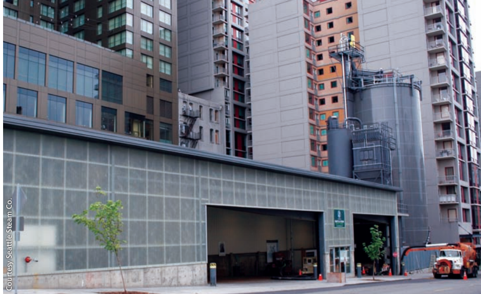
Seattle Steam’s new fuel handling facility is adjacent to one of its customers, the Four Seasons Hotel. The facility quickly took shape in 2009, with construction of the storage silo (right) attracting community attention. Uniquely, the roof section went up first, and the silo was built from the top down by jacking up each course of the tank over the eight-week construction time frame.
