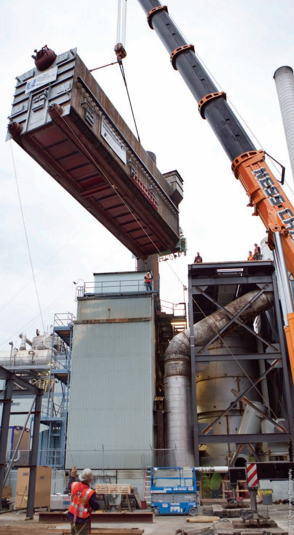
Seattle Steam Co. brought in the largest mobile crane in the Pacific Northwest to lift its new biomass-fired boiler into position at its Western Avenue Plant in downtown Seattle.
